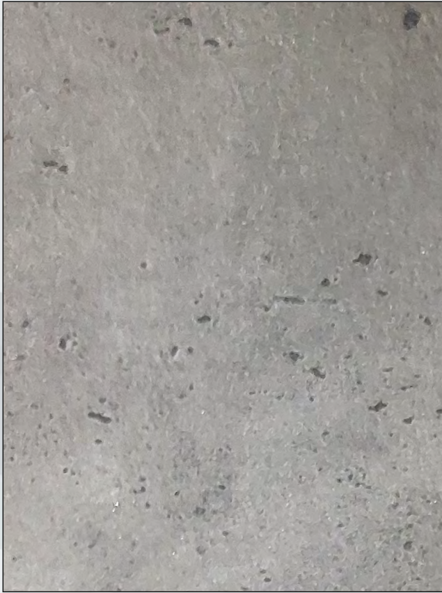
R-709 STX-SKYLINE CONCRETE
